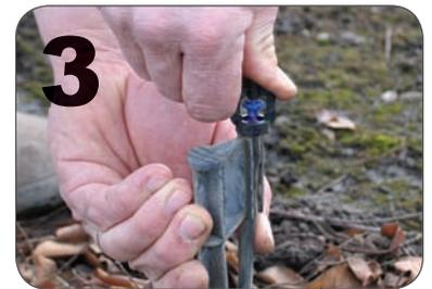
Install a new R5 Rotator (flush with the top of the existing stake). The flow of the new R5 nozzle should closely match that of the old micro-sprinkler. Consult with an irrigation dealer to obtain the flow performance of your old micro-sprinklers.
