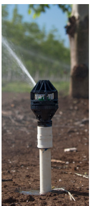
One of the most common methods of mounting an R2000 is on a PVC riser connected to an underground lateral line.
