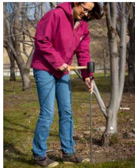
Use stake install tool 13429 to pre-make holes for the QC4 and QC5 stakes. This ensures that the stakes will be installed straight.
